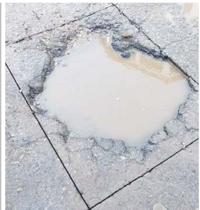
The Road Repair method used; where they cut around the pothole; cut it off and then pour tarmac and let motor vehicles press or compact it. A small roller also used at times. Repairs done at night!
